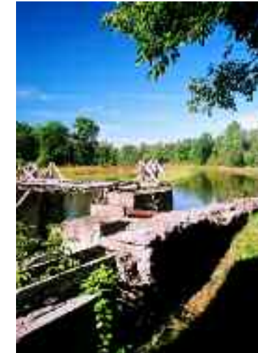
Stockdale Mill Dam
