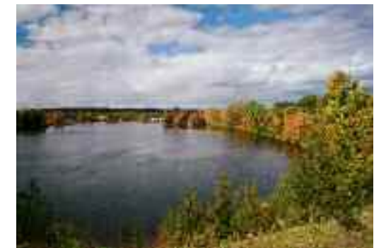
Trent River Dam - Quinte West
